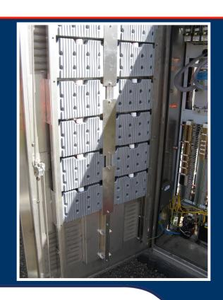
2. The introduction of temperature management blocks (TMB) into the interior of the enclosure to absorb the heat energy and store it.
