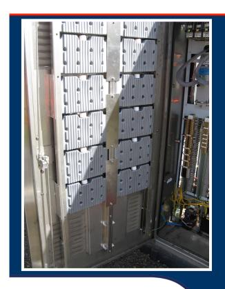
The Blocks contain a Phase Change Material – PCM27 PCM 34 & PCM46
