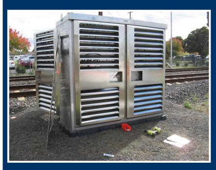
1. External enclosure panel fitment. Reducing the effects of the sun or Solar Gain, This can be as much as 1.5kw p/m2 and has an immediate impact on the internal ambient temperature.
